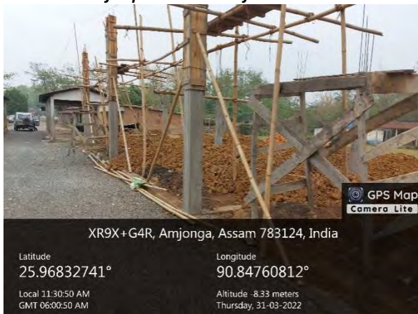
Working at height not properly adopted. Improper scaffolding
