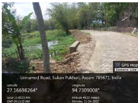
Earther Shoulder needs to be stabilized
