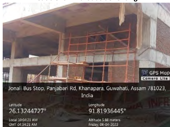
Working at height station not properly installed. Safety railing not installed
