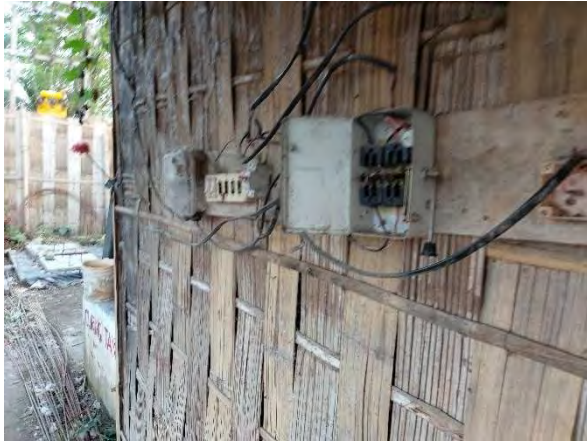
Loose wire and electric board on wooden wall of labour camps
