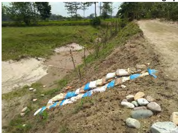
Sand Bags placed at the cross drain structure to prevent washing off of loose soil
