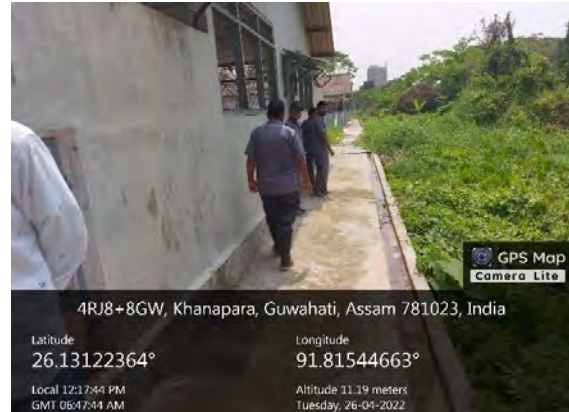
Lines drains noticed all along the sty. These drains leads into water ponds within plant premises.
