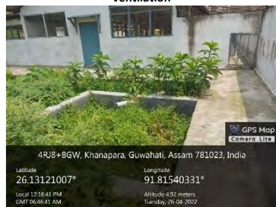
Soak pits silted, need de-silting on urgent bases.
