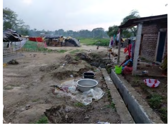
Construction of lined internal drains
