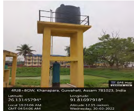
Over head tanks for water supply with pig farm. To maintain good quality of water, filter has been installed.
