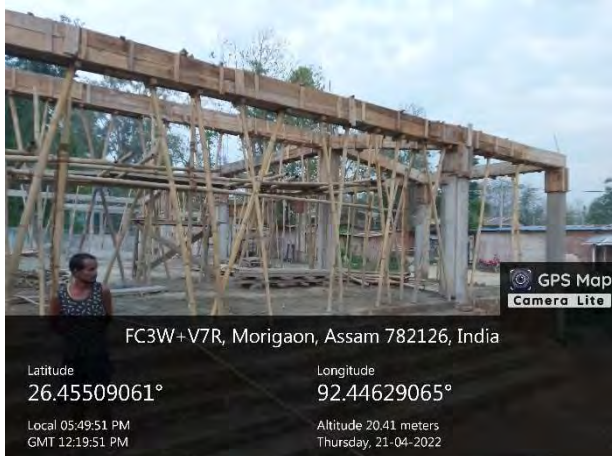
Scaffolding with timber at construction site
