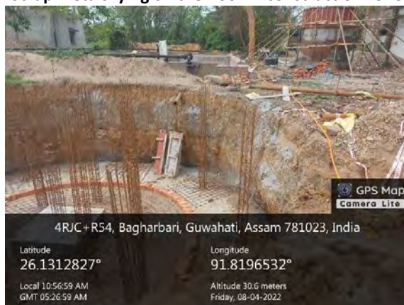
Cut trench without side fencing
