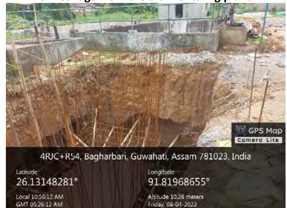
Cut trench wall collapse, hazard issues
