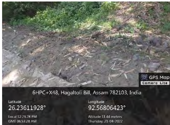
Earthen Shoulder washed off during Rain
