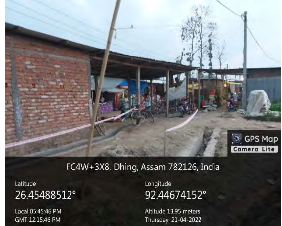
Safety strip at cut area for construction of drains
