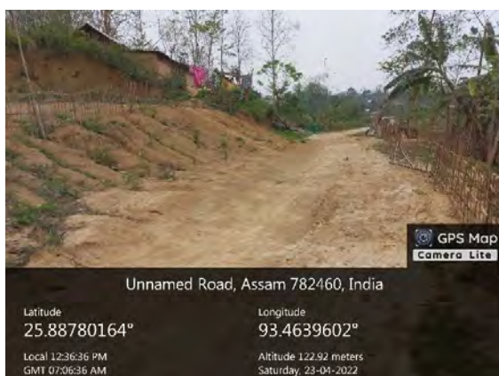
Road damaged due to cut soil reaching the ROW.
