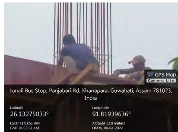
Worker working at height without safety belt
