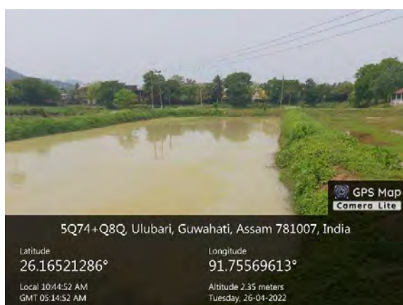
Vertical cut wall of the rearing ponds, needs slopy side wall
