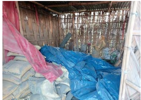
Stocking of cements bag on earthen surface
