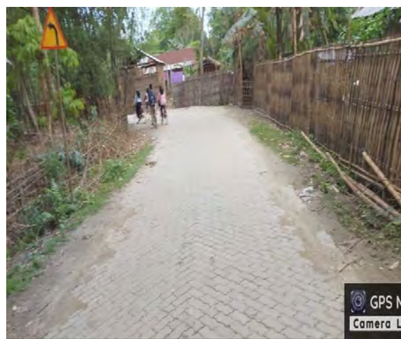
Pavers Block roads which are hard and eco-friendly
