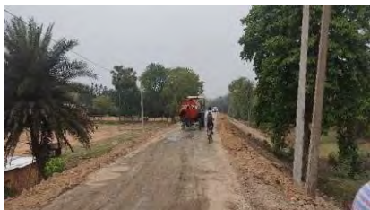
Water sprinkled for dust suppression
