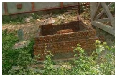
Underconstructed overhead tank & rainwater harvesting pit
