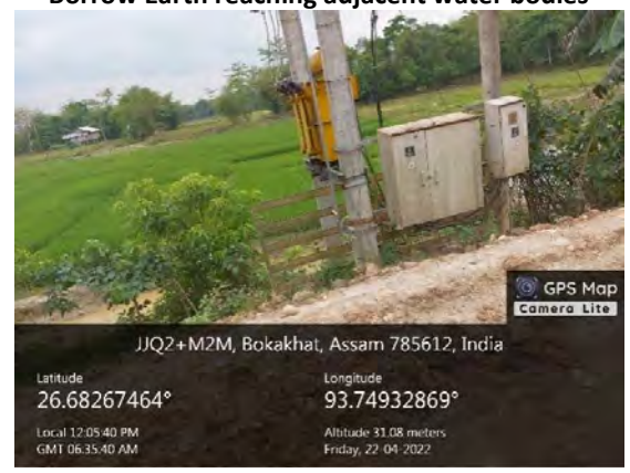
Borrow earth stacked at the transformer without maintaining safe distance
