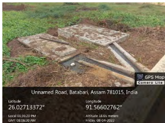
Soak pit and septic tanks over flowing pollution soil and nearby water bodies
