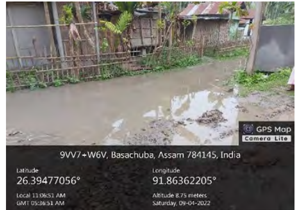
Flooding on path connecting the proposed road due to no cross drainage structure.
