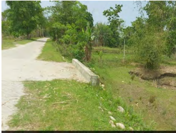
Cross drain structure and stone pitching to prevent cutting and erosion
