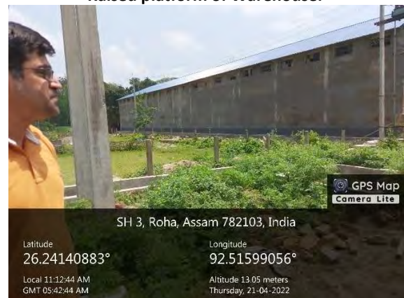
Roofing of warehouse meeting climate resilience specification. Very high roof to maintain internal cooling
